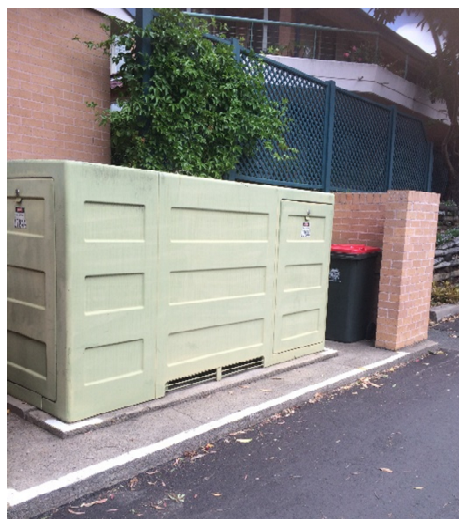
Figure 1 – Kiosk Substation
